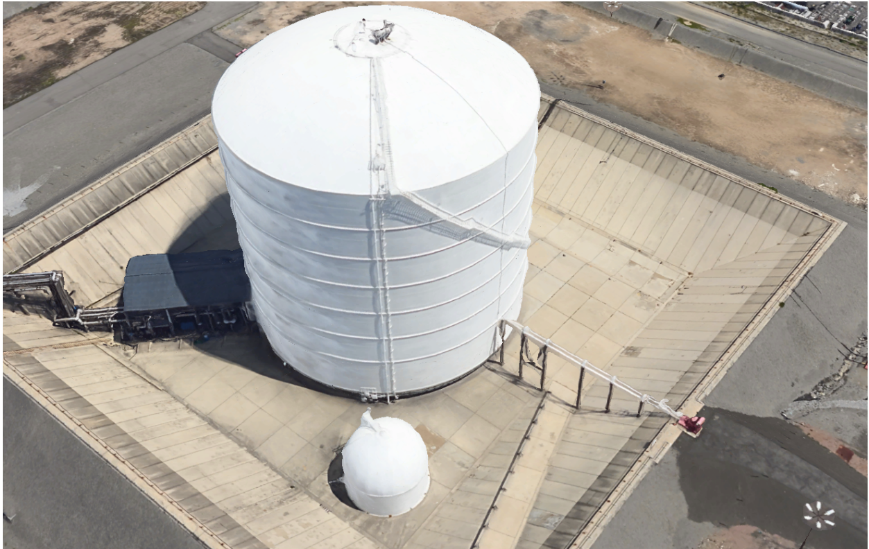
Figure 17: Google earth random picture a near atmospheric LNG tank
