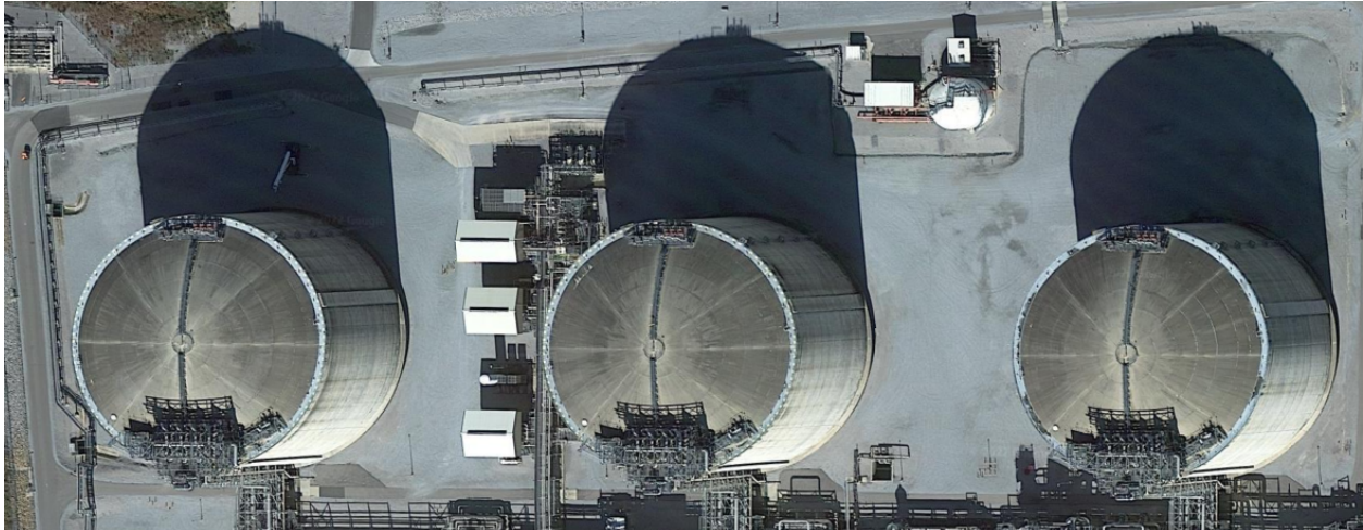
Figure 19: Three full containment LNG tanks
