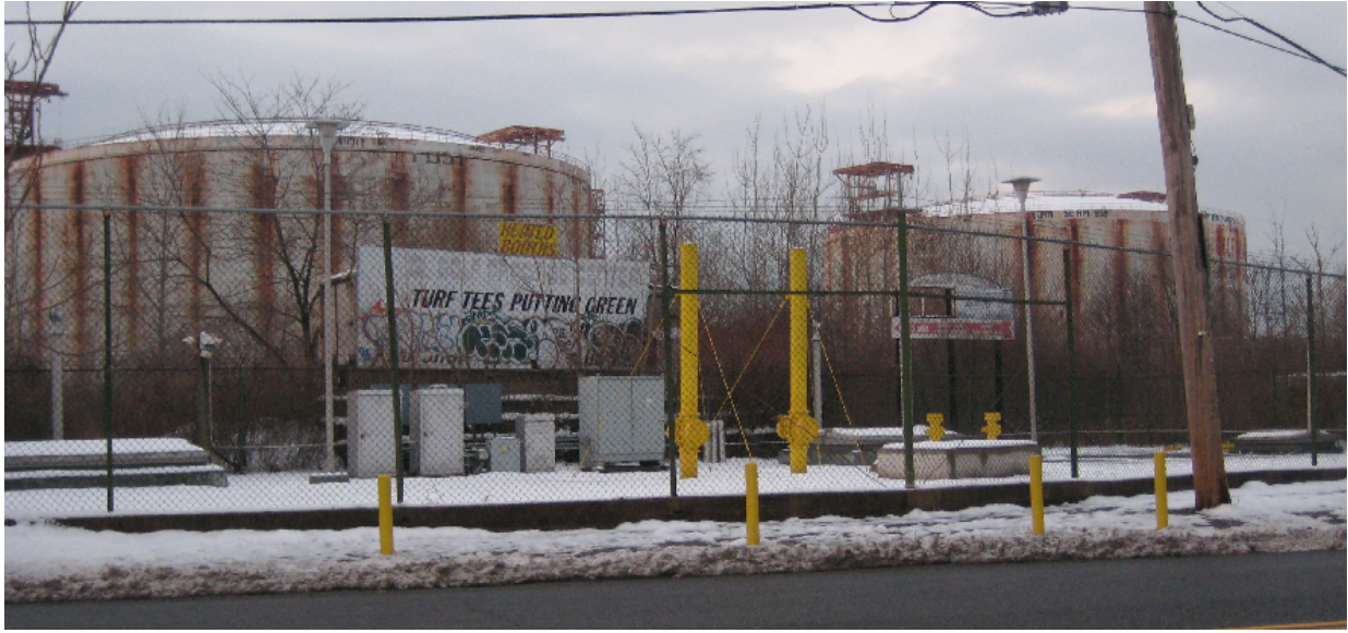
Figure 24: Two Full Containment LNG tanks that never saw a drop of LNG due to public and political opposition (built in early 70s).
